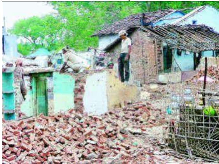
Houses in Harsud being demolished to discourage residents from returning.
